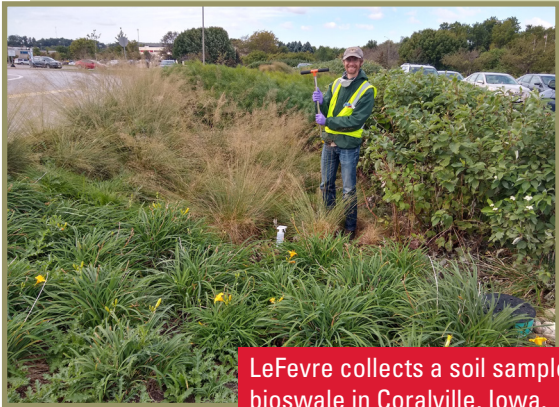
A Bioretention cell used to collect and infiltrate stormwater. Note the cut in the curb that collects stormwater and the use of native plants.
